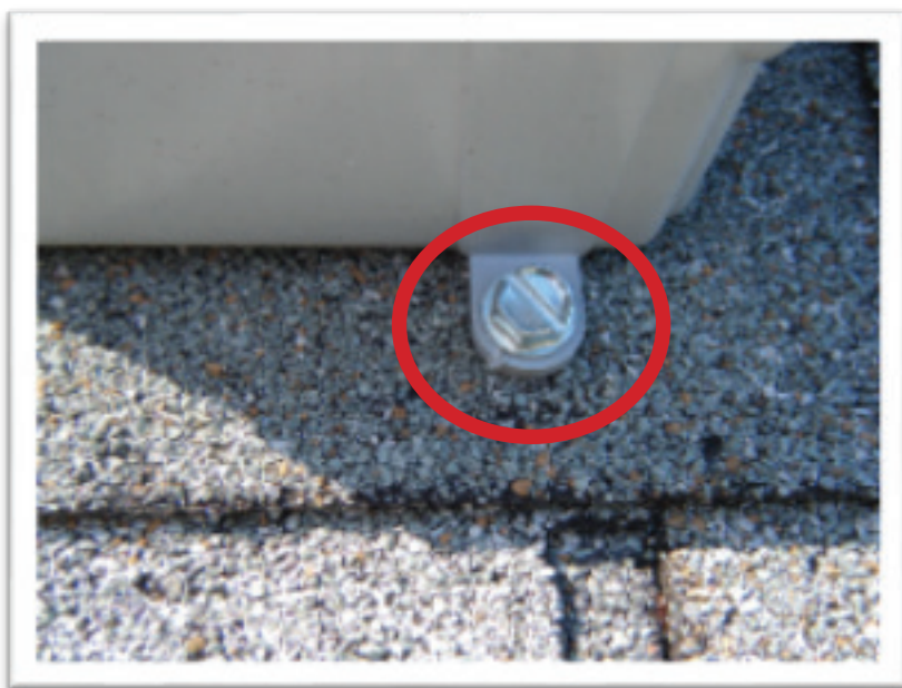
Photo D6: Roof penetrations and anchors not flashed: International Building Code 1503.2, International Residential Code 903.2.
