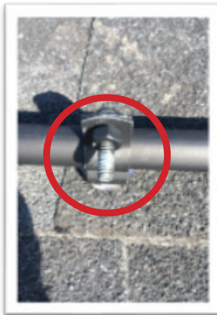
Photo D6: Roof penetrations and anchors not flashed: International Building Code 1503.2, International Residential Code 903.2.
